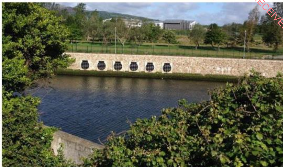
Figure 3-1 Culverts at Ravenswell Road (view from the right bank of the River Dargle)
